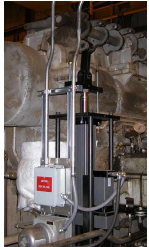
Figure 4. Electric Actuator direct on valve rack
