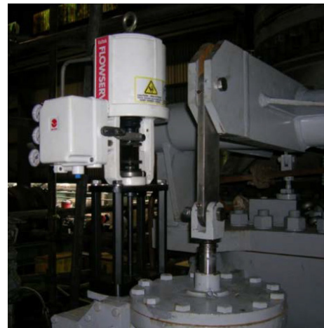
Figure 3 - Pneumatic Actuator on pilot operator power cylinder
