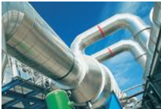
Honeywell's Experion® Process Knowledge System (PKS) includes a world class SCADA system that drives critical information to the pipelines operations team while automating data logging and processing.
