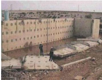
Collapse of new storm basin during first test, damage to hydrogen line with leak and site evacuation
