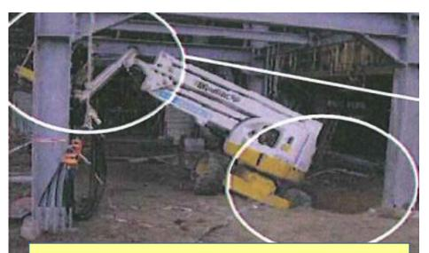
Worker died while moving persons lift from cabin using cabin arm as counterweight
