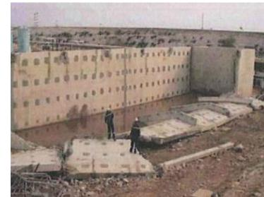
Collapse of new storm basin during first test, damage to hydrogen line with leak
