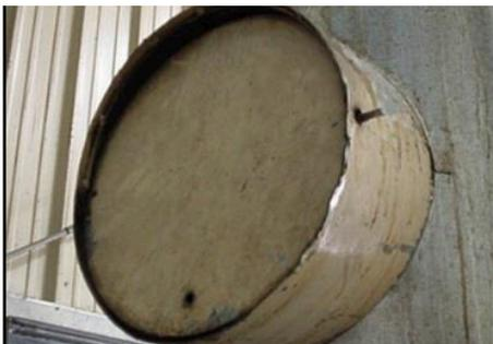
These devices consist of what looks like a loosely hung damper blade with some type of weight or adjustment.
