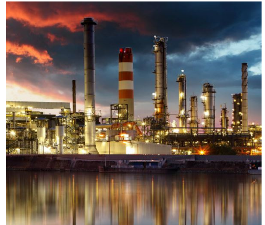
Total Care Lite is a cost-effective way to achieve regulatory compliance and improved reliability for terminal assets, with remote support for faster resolution of issues.
