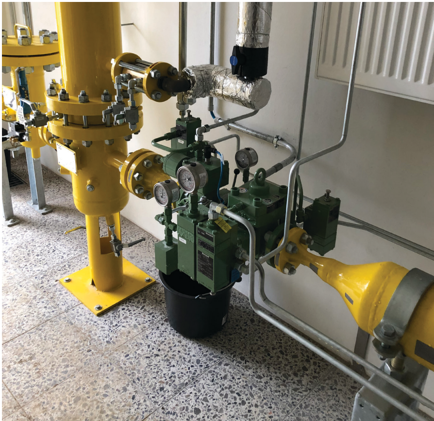
Gas pressure reducing station "Wittenborn"
