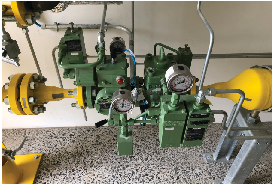
Gas pressure reducing station "Witzwort"
