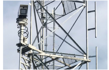
Hardware monitoring devices installed.
