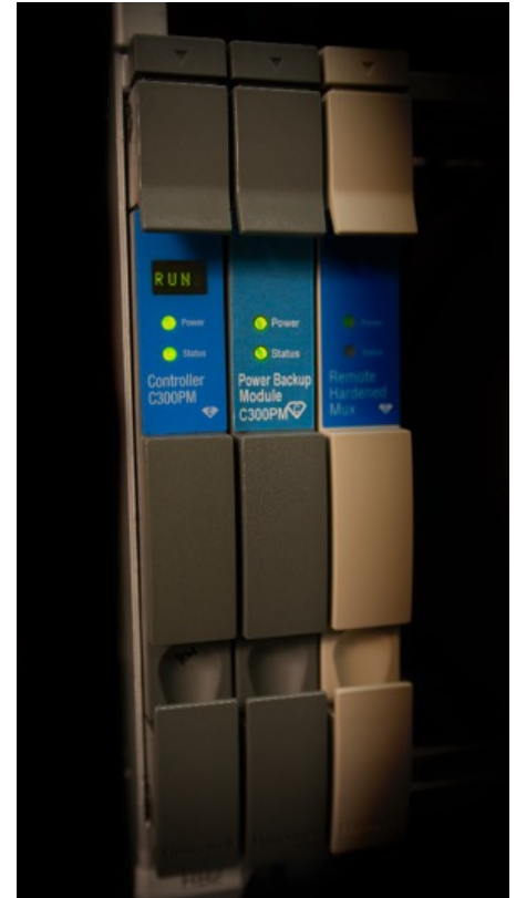
Figure 3: The C300PM combines the features of the EHPM and C300 in an EHPM form factor.
