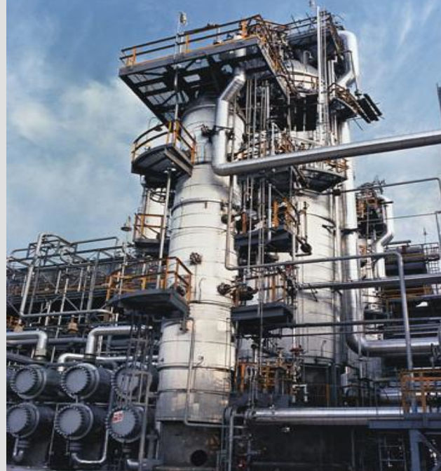
Refinery Revamp of Existing Hydrotreater
