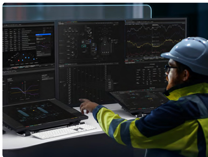
Figure 2: Experion Operations Assistant leverages machine learning to predict near-term events and anomalies and offer guidance within the Panel Operators workstation.
