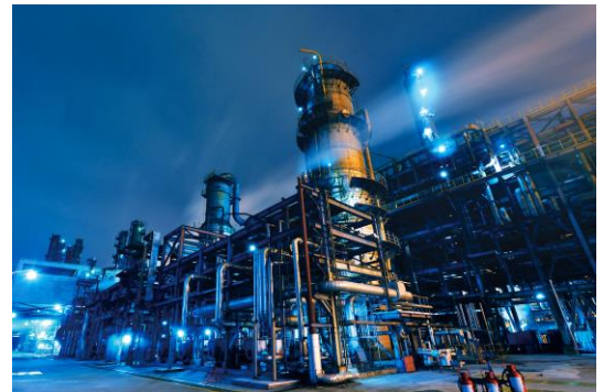
The Honeywell PCN Hardening service is a driver of improved compliance and safety at today's industrial facilities. Expert industrial cybersecurity consultants carefully evaluate, customize and enforce cybersecurity recommendations for process control installations.
